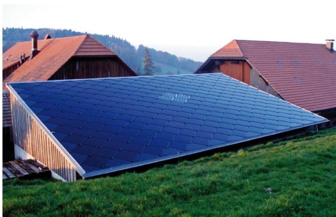
Figure 3: Diamond shaped solar tiles
