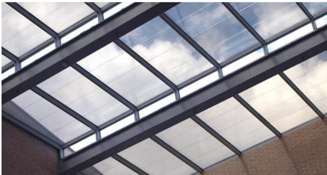
Figure 5: Transparent solar PV cells
