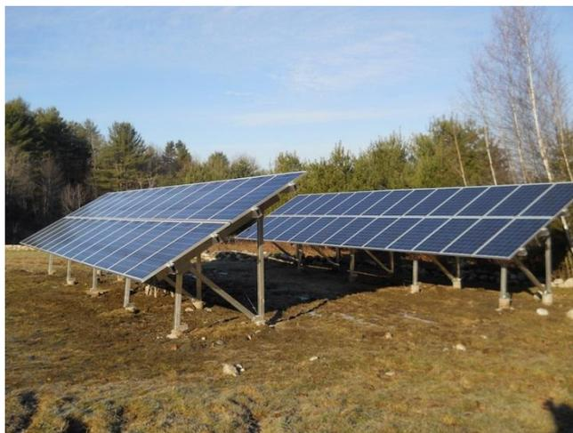
Figure 12: Ground mounted solar PV system
