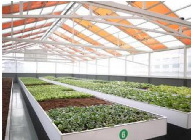
Figure 6: Coloured solar cells
